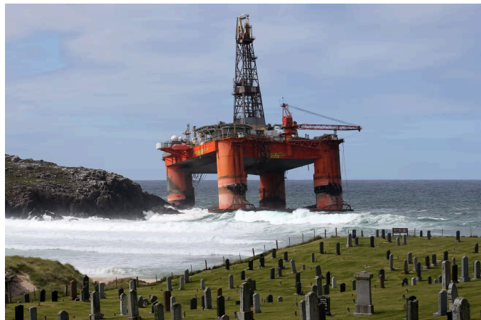
decommissioned oil rig running aground off the coast of the Isle of Lewis
